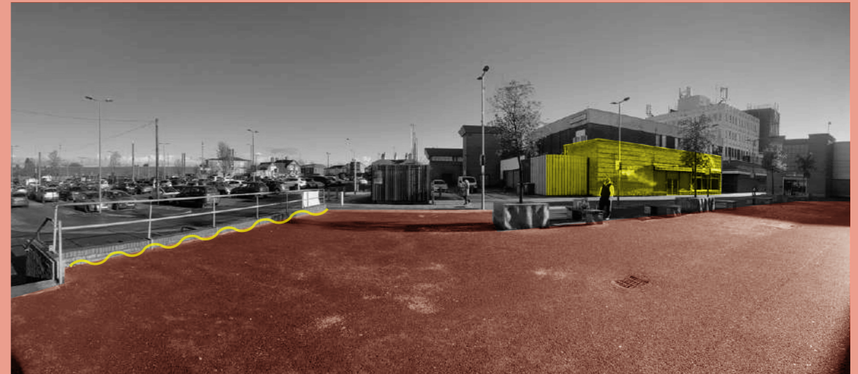
Sparse planting and unattractive macadam surface, defined by empty retail units does not create a welcoming or safe place to dwell or relax
