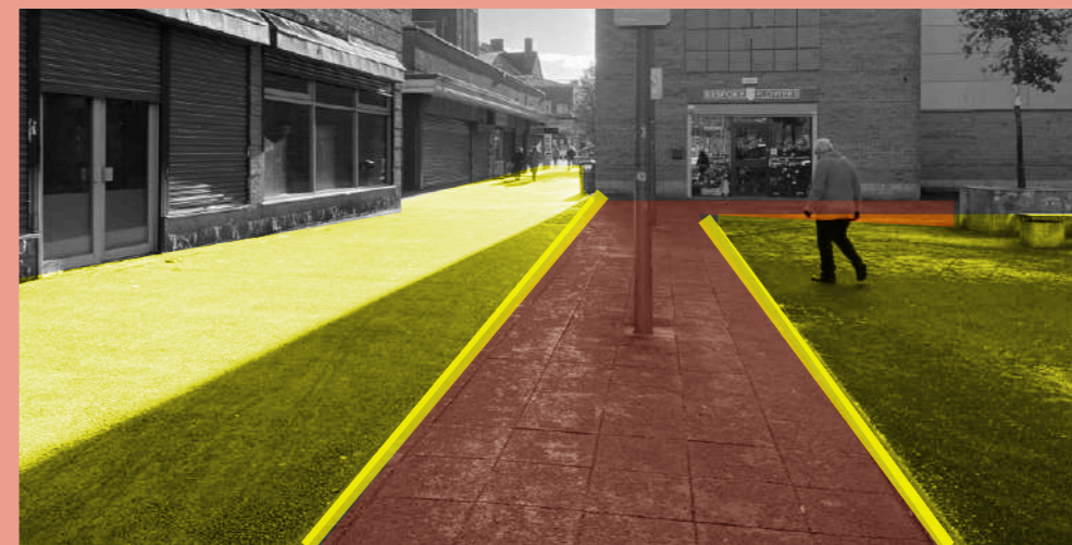
Patchwork of hard surfacing materials creates a disjointed environment that appears tired and vacant
