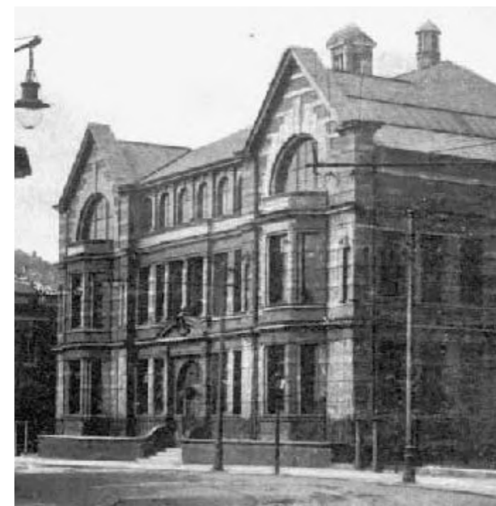
Technical School, Stalybridge
