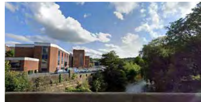
8 Portland Place - View South
