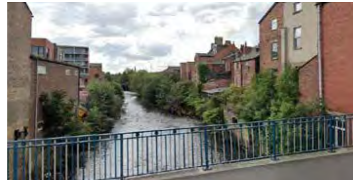
2 Melbourne Street Bridge - View West
