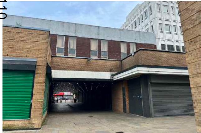
Voids within the buildings
