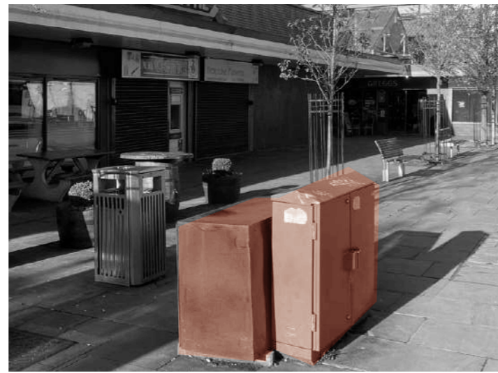
Cluttered, poorly laid out infrastructure
