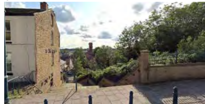
4 King Street Steps - View South
