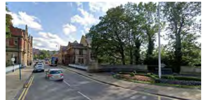
12 Portland Place - View South
