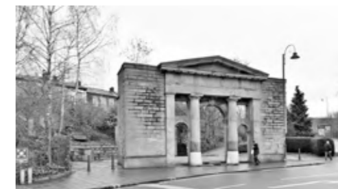
B Former Town Hall | Grade 2 Listing 1831
